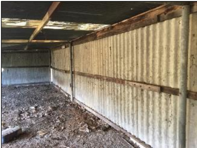
Plate 29 – ACM cladding in rear shed.
