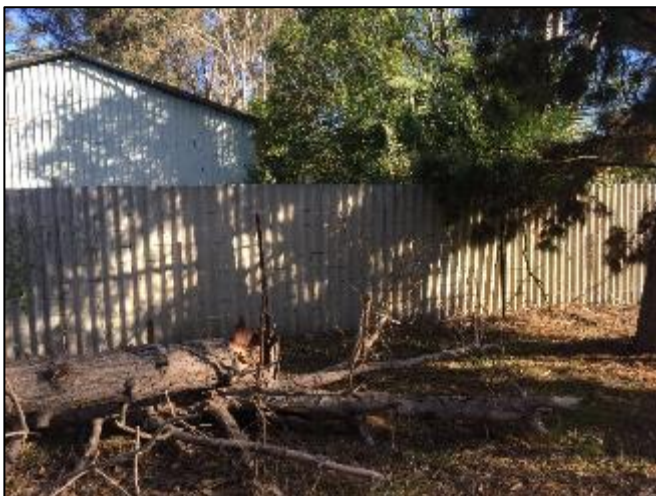
Plate 11 – View towards the large shed showing ACM clad fence.
