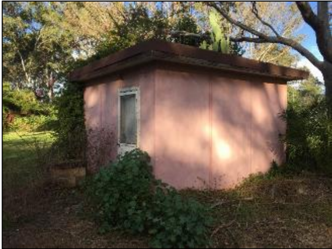
Plate 7 – ACM clad external laundry
