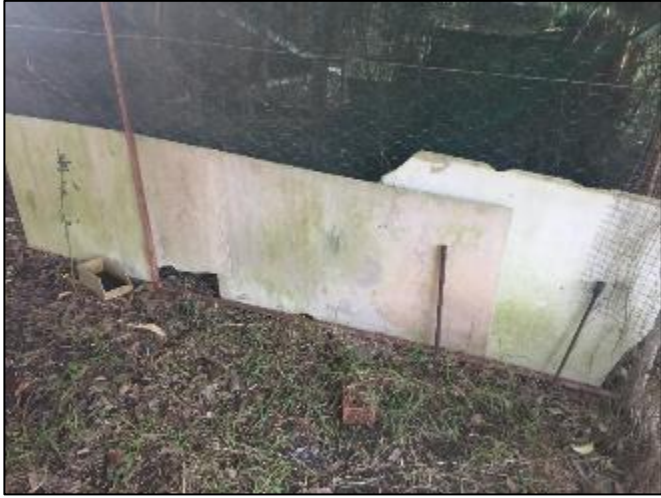
Plate 31 – ACM sheet used to patch fencing in the kennels.
