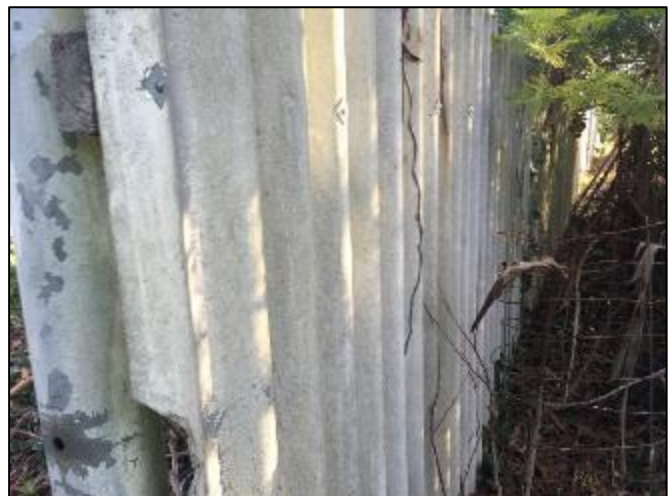
Plate 12 – ACM clad fence in the central portion of the site in moderate condition.
