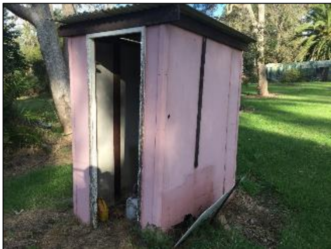
Plate 6 – ACM clad external outhouse.
