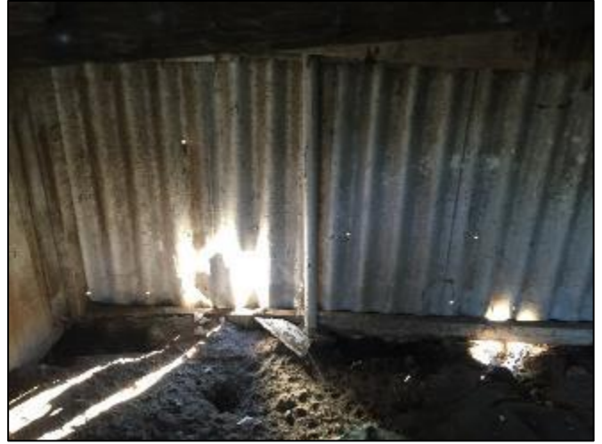
Plate 32 – Broken ACM cladding in kennels subject to partial burial.
